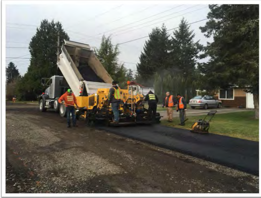
Paving on Brunswick Street SE (April 2018)
