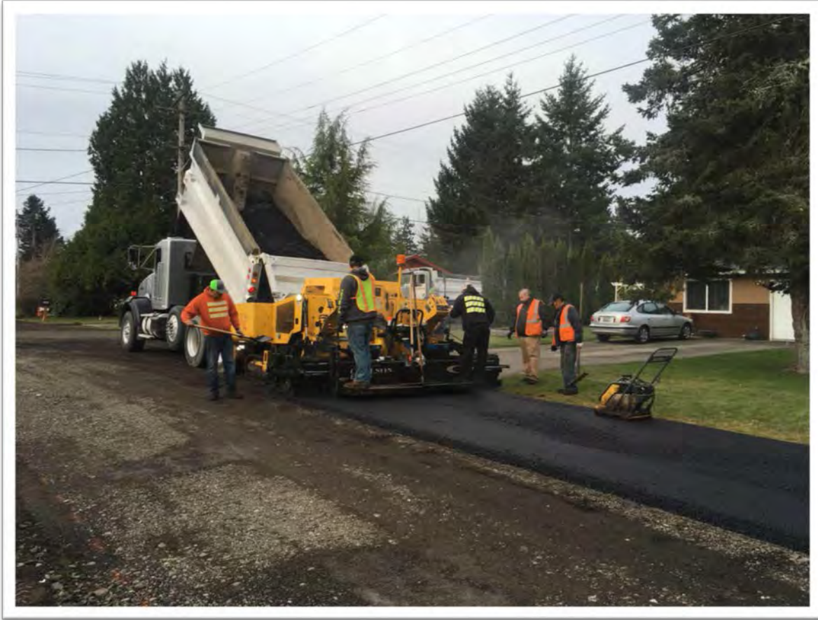
Paving on Brunswick Street SE (April 2018)
